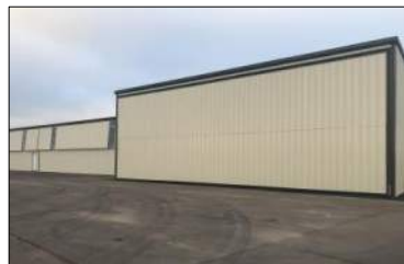
T-hangar with Large End Bay
